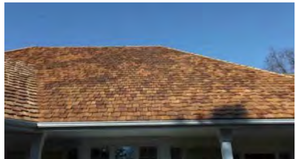
Figure 28: Wood Shakes
