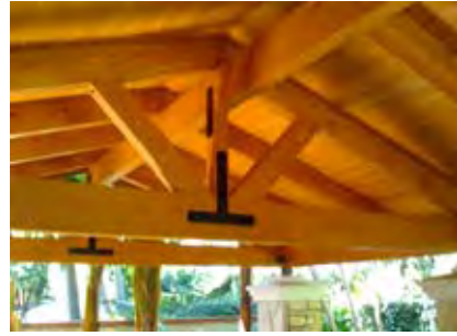
Figure 10: Type IV Construction
