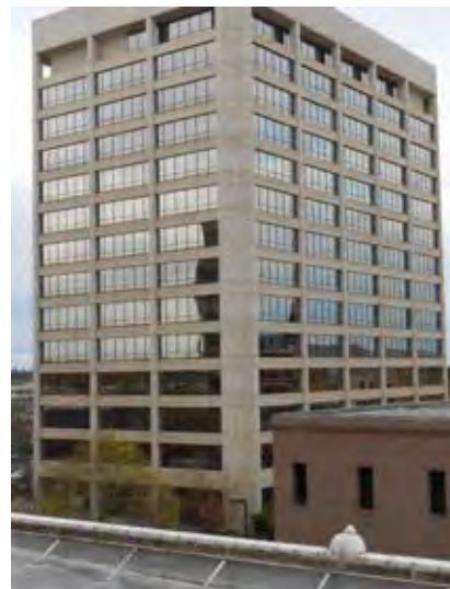
Figure 12: Type I Construction
