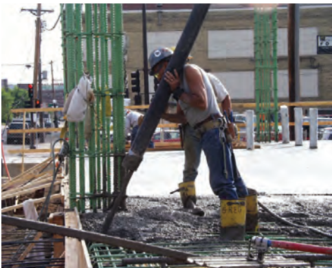
Figure 24: Placing Concrete
