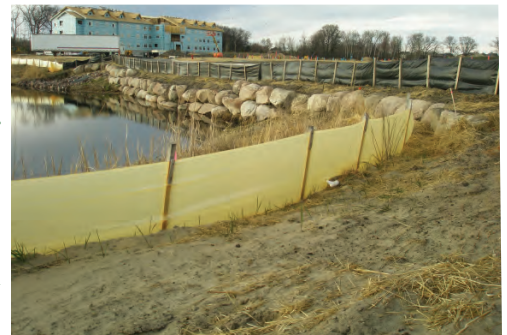
Figure 6: Soil Erosion Control
