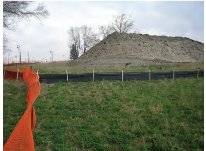
Figure 14: Stockpiled Excavation Material
