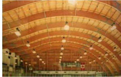
Figure 16: Heavy Timber Construction
