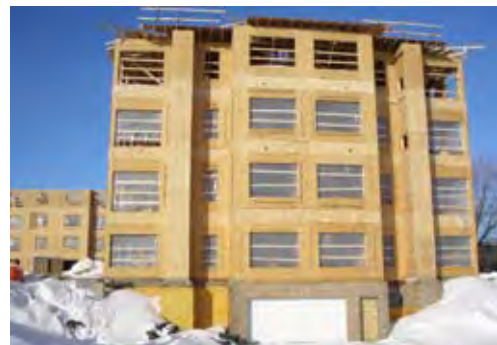
Figure 9: Type V Construction
